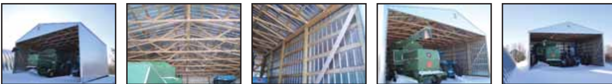
32'x32' pole shed, open on one end.
