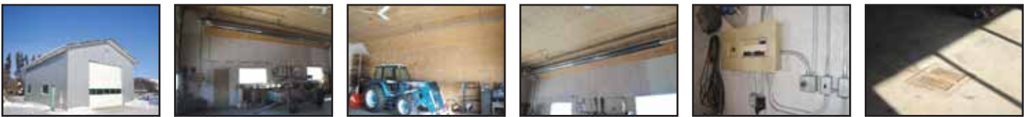
30'x40'x16' heated shop with 14H'x16W' door, concrete floor.
